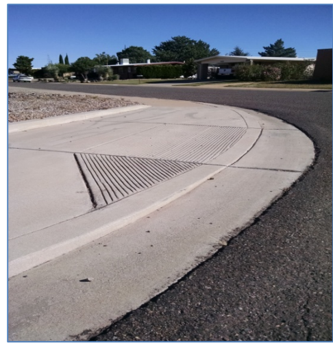
Meets: Graded indicator lines, flush
